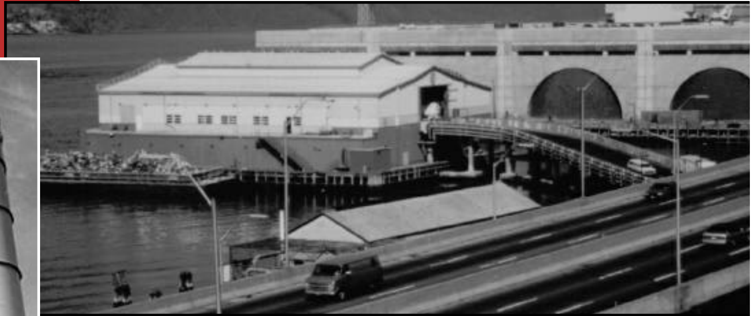
Current conditions at the Harlem Piers
